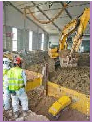
Soil excavation and the use of slide rail shoring.
