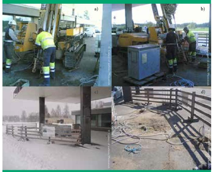
From a-d : a) Jalasjärvi site, b) the installation of perforated tubes and c), d) the electrokinetic in situ treatment.
