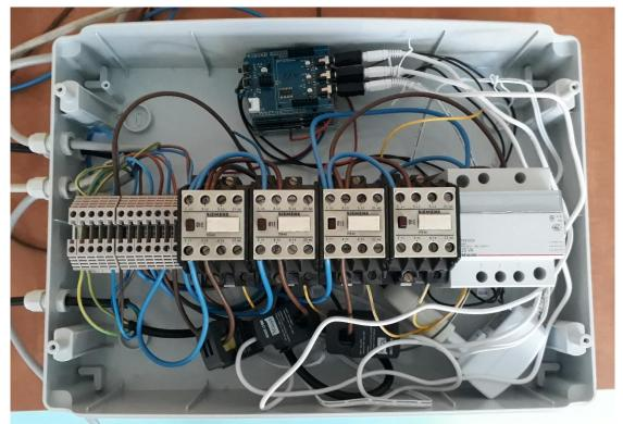
Figure 20. Electric panel with metering and interconnecting devices
