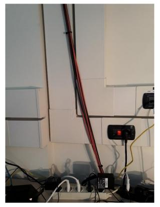
Figure 10. DC cables coming from solar panels on the roof of the building
