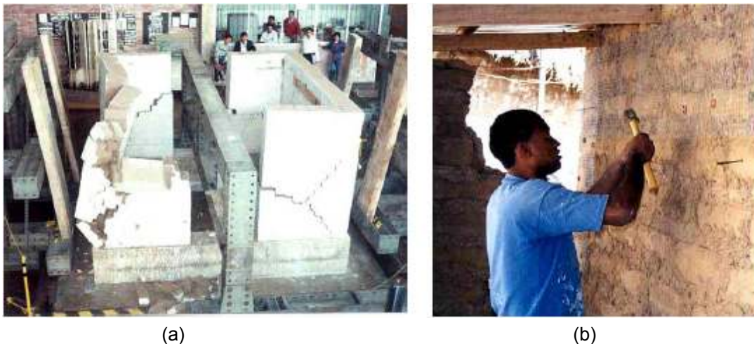
Fig. 4-14 (a) U Walls with and without mesh; (b) Wall wire mesh reinforcement.
