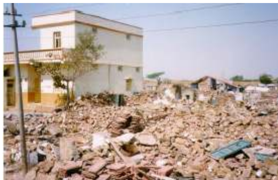
Fig. 4-50 Residential building constructed using brick masonry with lintel band survived at Ratnal. (source: IITB and EDM/NIED, 2001)
