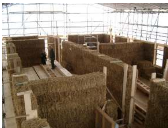
Fig. 3-34 Straw-bale house under construction.
