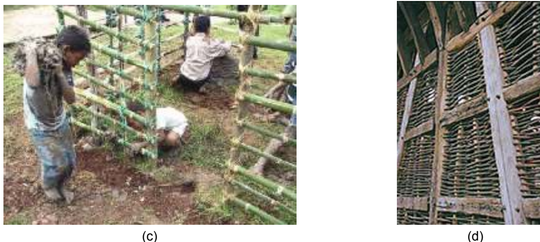
Fig. 3-35 (a) A wattle and daub building in Cayman Islands; (b) Traditional wattle and daub system, Venezuela; (c) Quincha building tutorial in Panama; and (d) Panel to be in-filled with earth. [sources: (a) http://www.cayman500.ky/img/ACF14E6.pdf ]; (b) Minke, 2001; (c) photo by Barkema, D. in http://www.thepanamanews.com/pn/v_09/issue_13/community_01.html ; and (d) http://www.northcoast.com/~tms/papercrete.html ]
