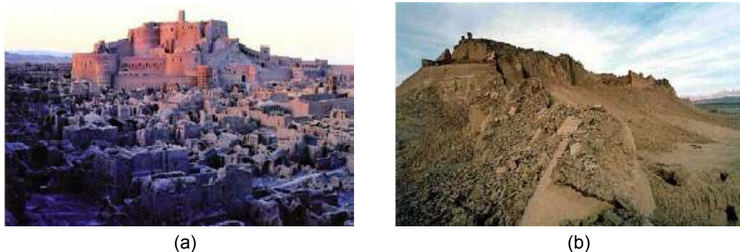
Fig. 4-8 The citadel in Bam: (a) before and (b) after the earthquake of December 2003. (source: Schroeder, 2004, "Building with Earth in Iran", available in: http://www.dachverband-lehm.de/pdf/DVL_terra2003_bam_gb.pdf )
