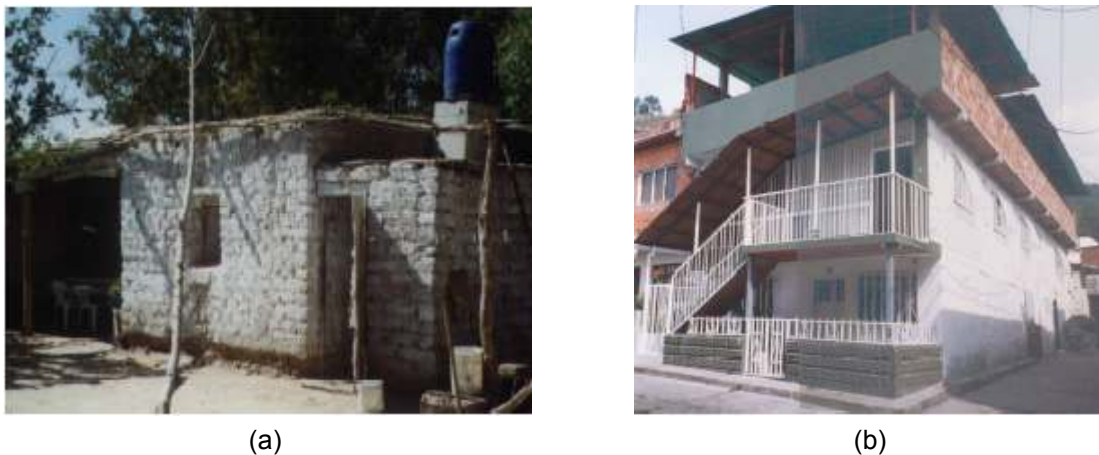
Fig. 1-12 (a) Traditional adobe dwelling in Argentina; (b) Non-engineered reinforced concrete frame building in Venezuela. [sources: (a) EERI, 2003; (b) EERI, 2002]
