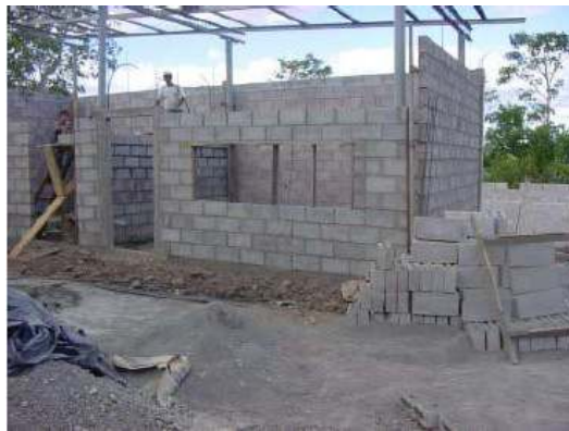
Fig. 4-26 Reinforced masonry house with concrete blocks under construction.
