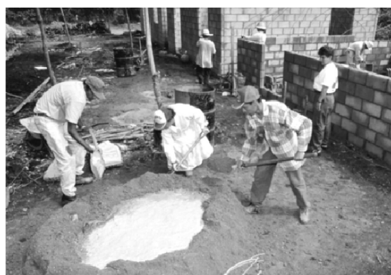
Fig. 2-2 Future homeowners work on their house in El Salvador. 7 (source: basin news / June 2002 / No. 23 : http://www.skat-foundation.org/resources/downloads/pdf/as/basinnews_23.pdf )
