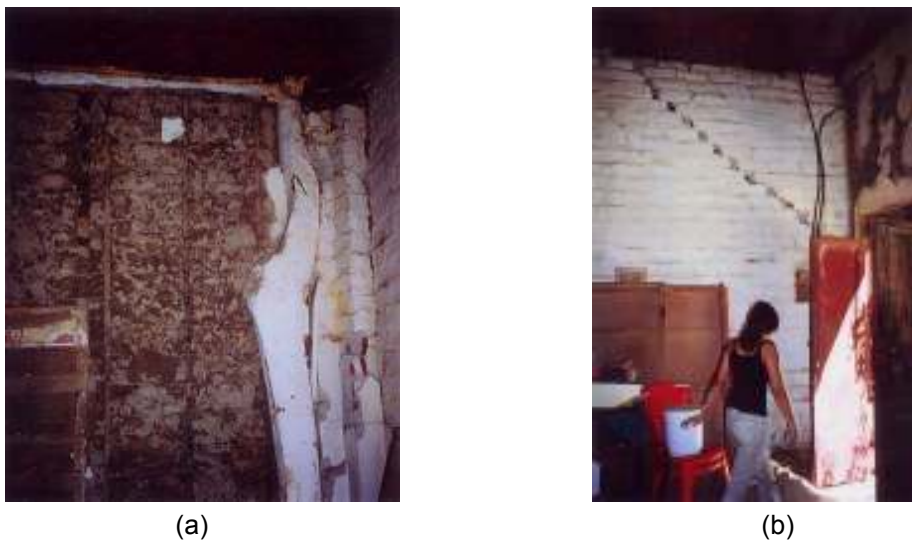
Fig. 4-47 (a) Adobe house with columns still standing in Verapaz; (b) Mixto house in Verapaz still standing next to an adobe house in total ruins. (source: photo by Manuel López Menjívar, University of El Salvador – annotated picture from EERI special newsletter report on the El Salvador earthquakes of 13 January and 13 February, 2001)
