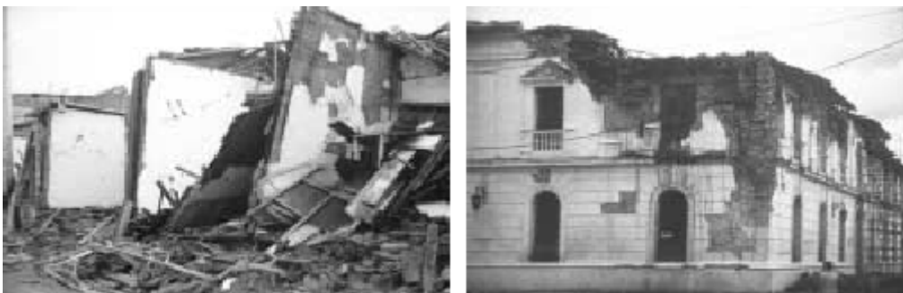
Fig. 4-6 Severely damaged rammed earth (“ tapiá ”) and bahareque dwellings. (source: AIS, 2002)
