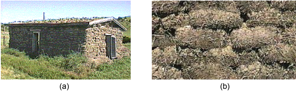
Fig. 3-27 (a) A “soddie” house; (b) Wall detail.
