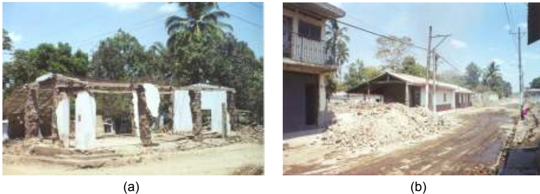
Fig. 4-47 (a) Adobe house with columns still standing in Verapaz; (b) Mixto house in Verapaz still standing next to an adobe house in total ruins. (source: photo by Manuel López Menjívar, University of El Salvador – annotated picture from EERI special newsletter report on the El Salvador earthquakes of 13 January and 13 February, 2001)
