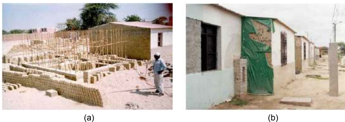
Fig. 4-13 (a) Cane reinforcement; (b) Finished dwellings after El Niño.
