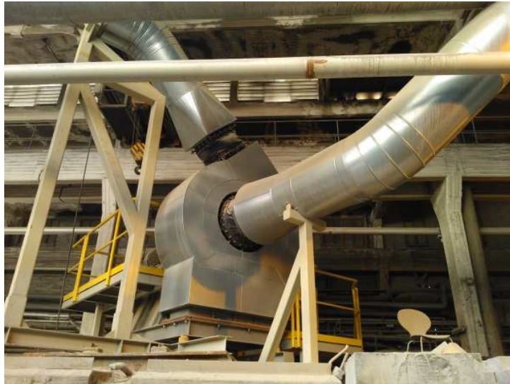
Fig. 3. Case study radial fan responsible for transfer of heat gasses from the cement kiln to the coal mill.
