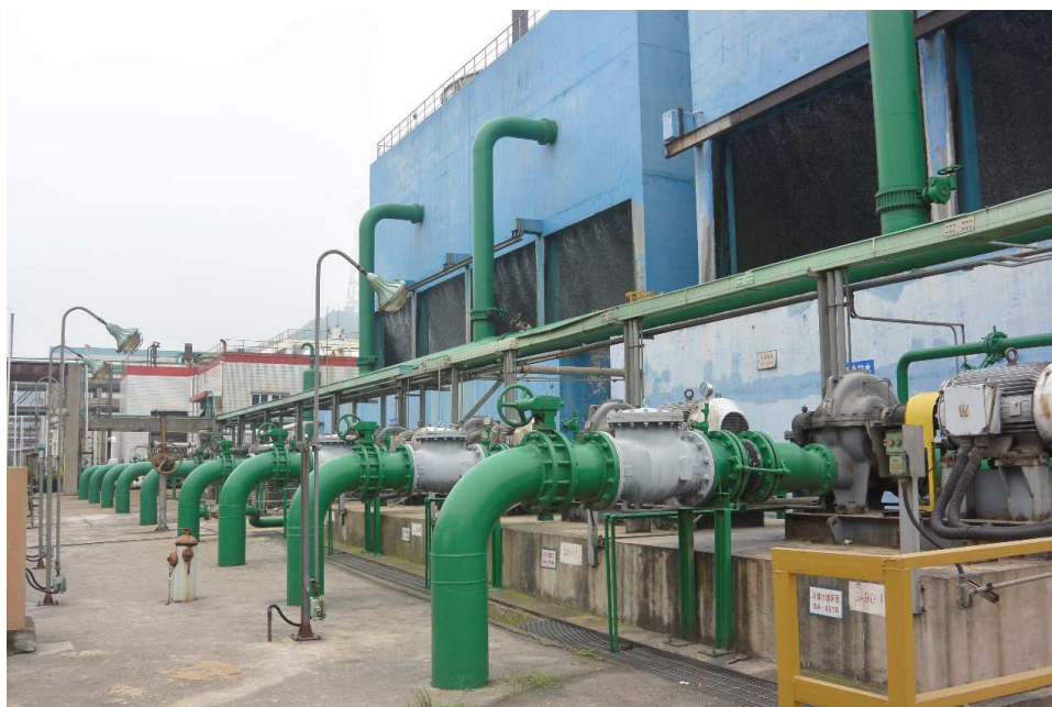
Figure 2 Circulating cooling pump system of pilot chemical factory
