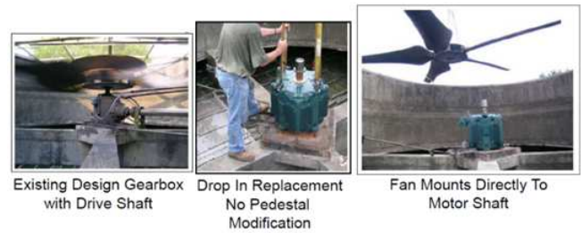
Fig. 1 Geared and gearless installations for cooling tower applications [1]
