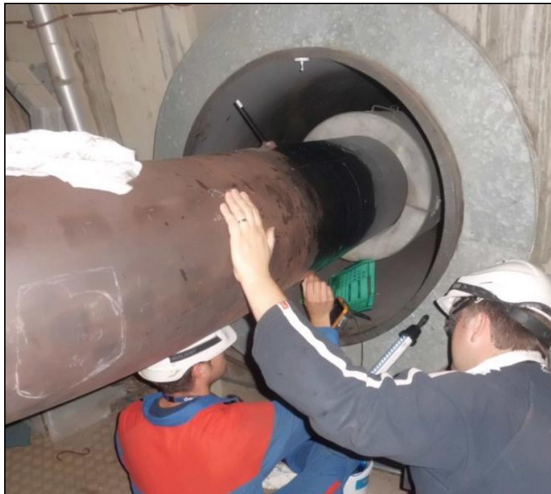
Figure 4. Example of manual UT test performed in a rather awkward position
