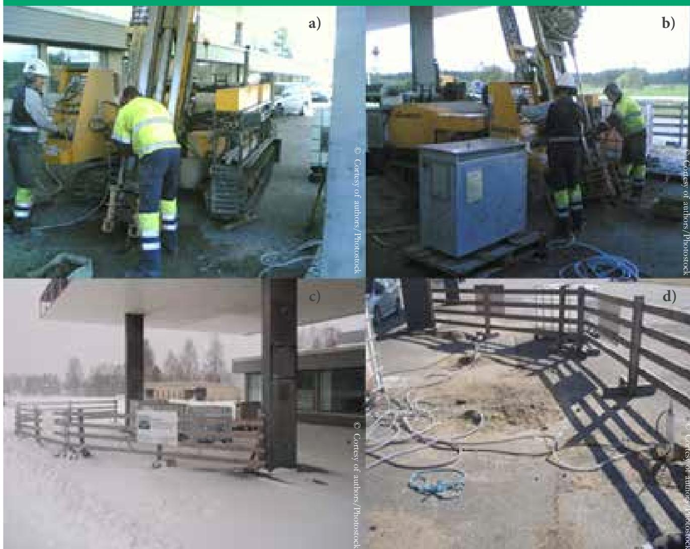
From a-d : **a)** Jalasjärvi site, **b)** the installation of perforated tubes and **c), d)** the electrokinetic in situ treatment.
