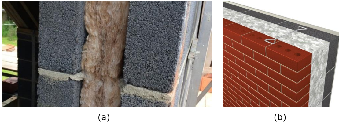
Figure 2.7 Typical Cavity walls in new buildings: (a) Detail of the insulation material; (b) Mechanical connection of the wall faces.
