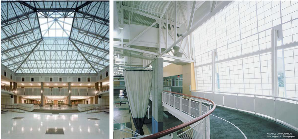
Figure 3.17 Two examples of translucent aerogel insulation as a high performance thermal insulation solution for daylighting; Source [69].
