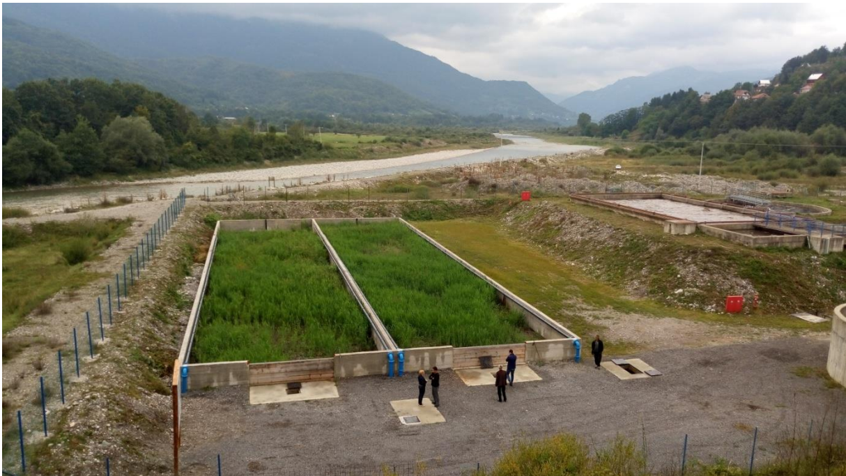
Figure 21 - Constructed wetland for sludge treatment in Mojkovac (Courtesy Alenka Mubi Zalaznik)
