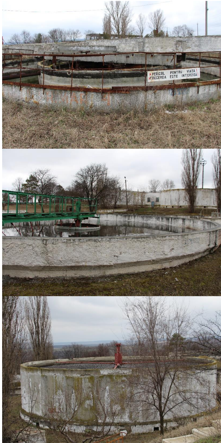
Figure 20 – views of the pre-existing, obsolete WWTP in Orehi, Moldova (courtesy C.Nanu)
