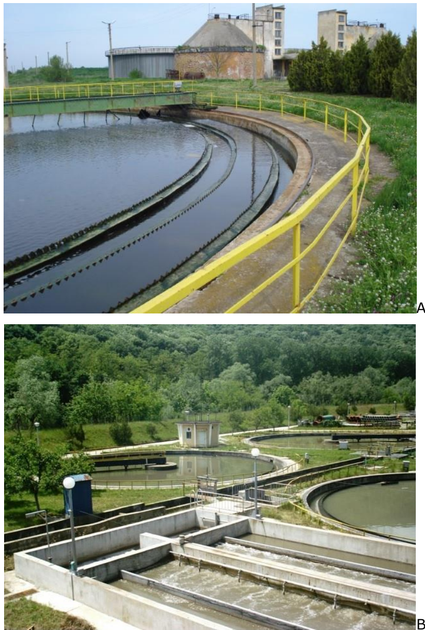
Figure 14 – View of the Razgrad (A) and Veliko Tarnovo (B) WWTPs. Courtesy C.Dimitrova.
