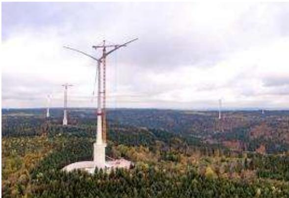
Figure 4 Gaildorf wind farm featuring four turbines with up to 178-m hub height.
