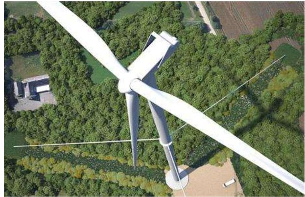
Figure 3 Artistic impression of a cable-stayed tower.
