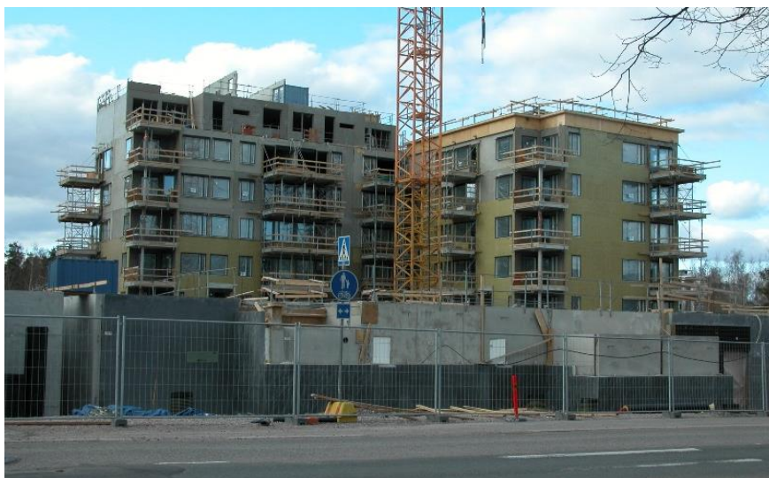
Figure 1. Construction using prefabricated concrete panels in Espoo, Finland (2010).
