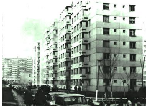
Figure 17. Typical 9-story precast large panel block of flats built in Bucharest since 1973.
