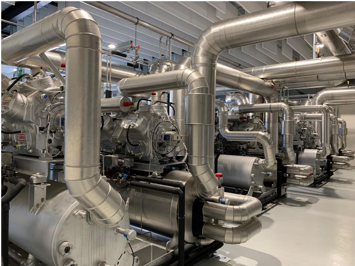
Figure 115: Heat pumps in Taarnby DHC network (source: Taarnby Forsyning )
