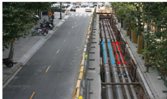
Figure 69: Illustration of the network supply and return pipes for DC (larger diameter, in blue) and for DH (smaller diameter, in red)
