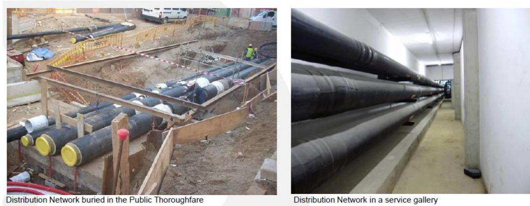
Figure 72: DHC pipes in multi-service public galleries (right), and in the public thoroughfare (left)
