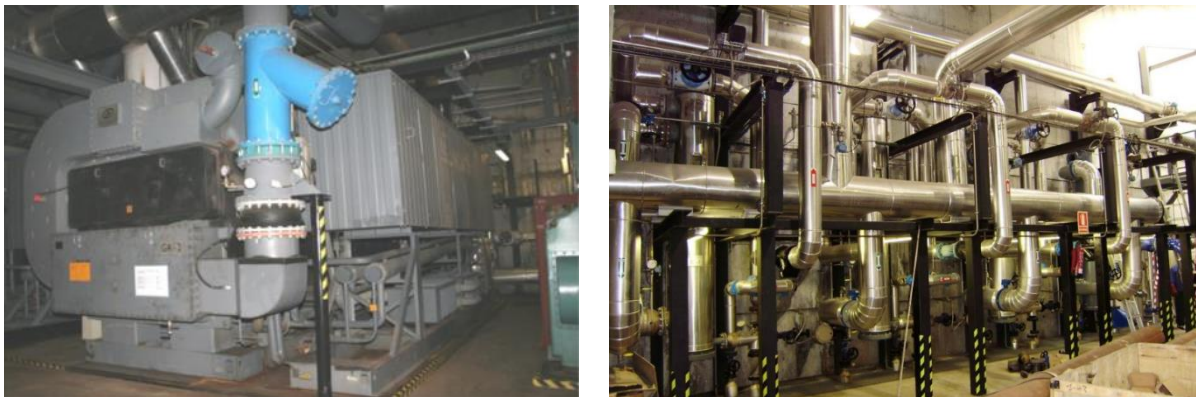
Figure 71: Broad absorption heat pump (left picture) and steam-water exchangers (right) in Forum plant (source: Districlima)
