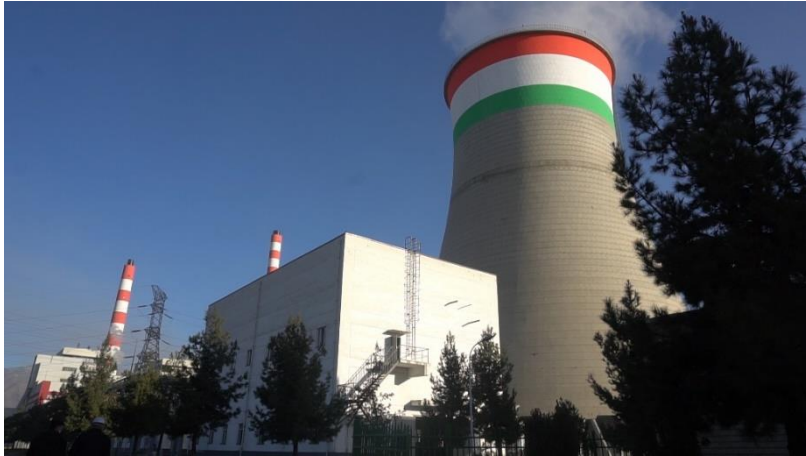
Figure 4. The Dushanbe-2 CHPP
