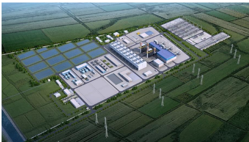
Figure 13. Sirdarya CCGT power plant outlook
