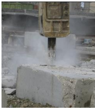
Fragmentation of a large reinforced concrete element
