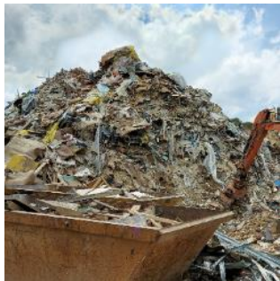
Removed materials from mixed CDW (preliminary sorting)
