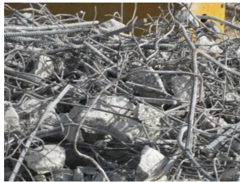
Reinforcement steel removed from concrete for recycling
