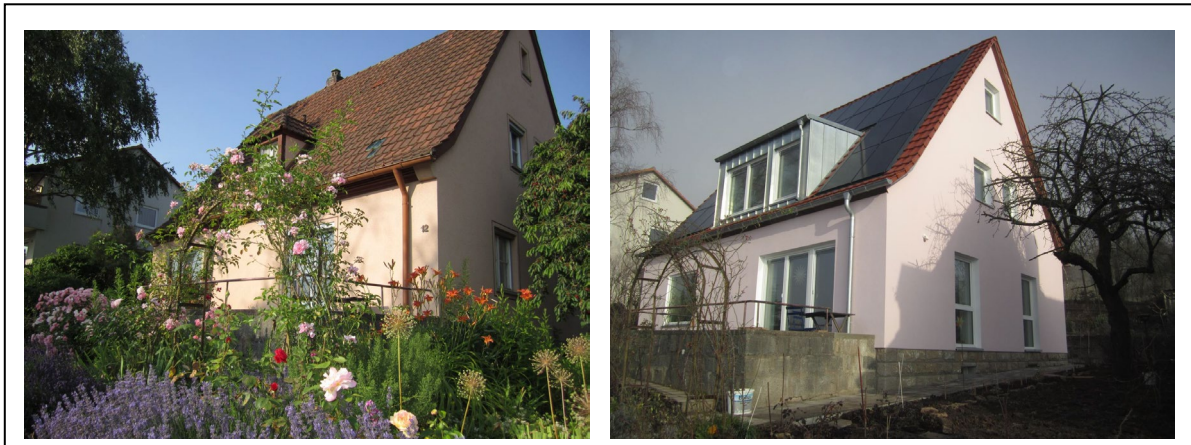
Figure 1. Building view (left photo - before renovation; right photo - after renovation)
