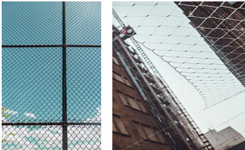
Figure 24: Examples of anti-drone fence (left) and stainless-steel net (right) deployed solutions
