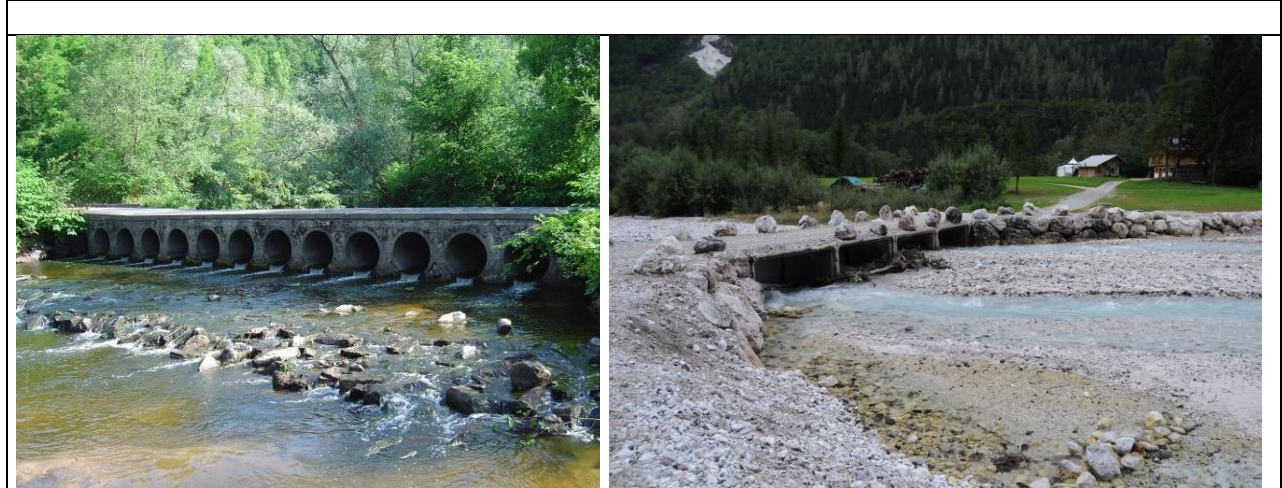
Round (left) and box-shaped (right) culverts
