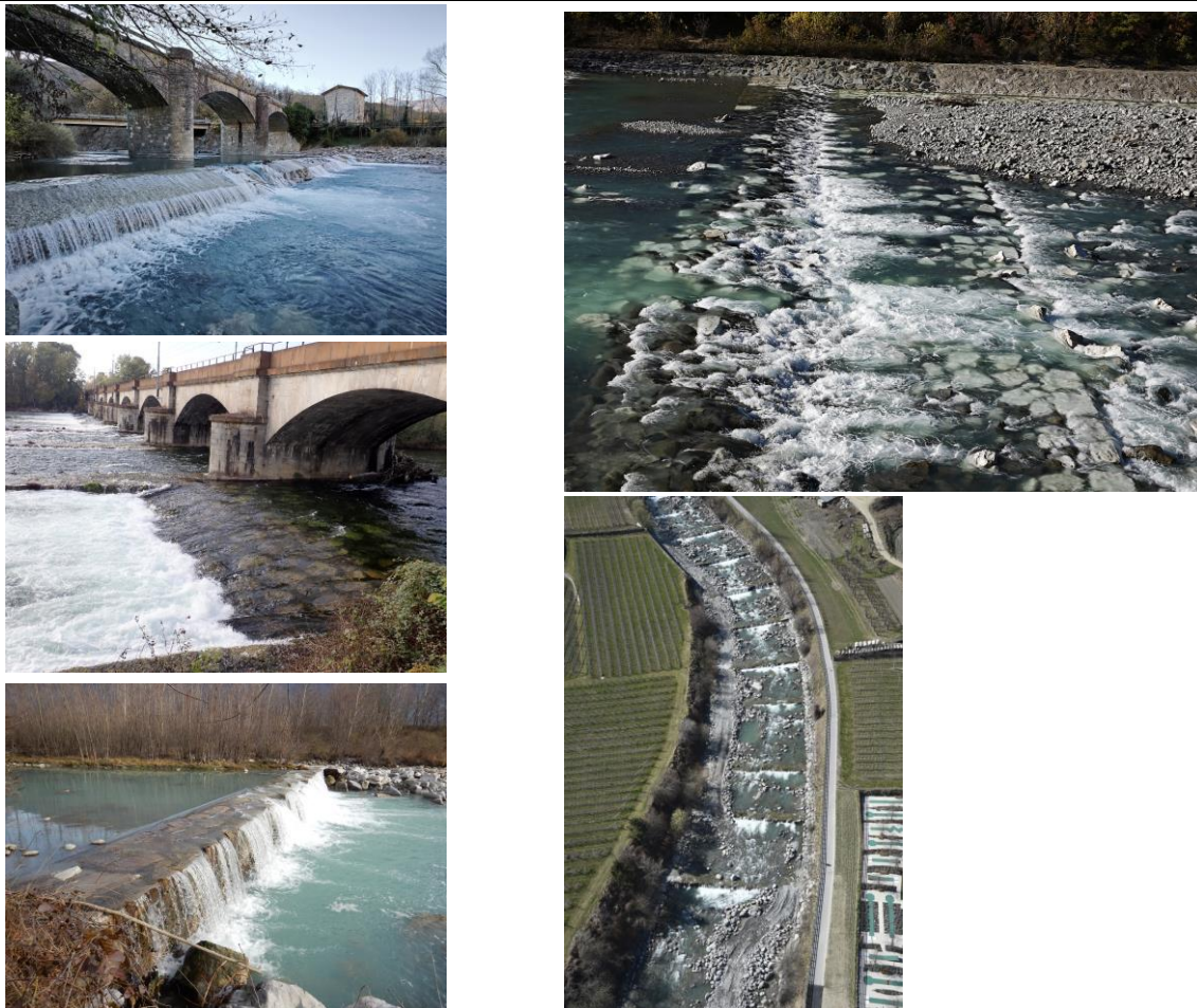
Left column: (top and middle) bed sills associated with a bridge; (bottom) bed sill
