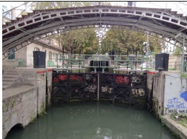
Lock gate for navigation
