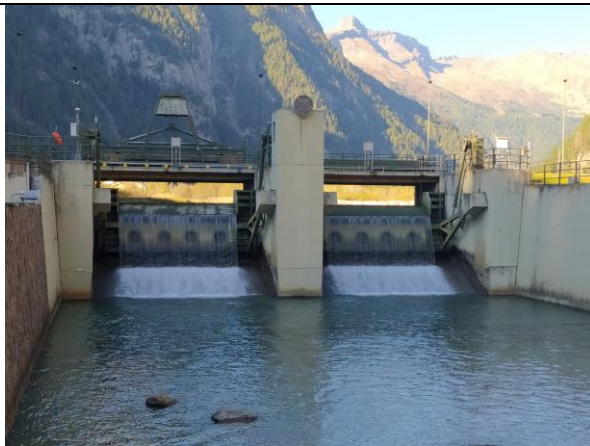
Sluice associated with an abstraction work
