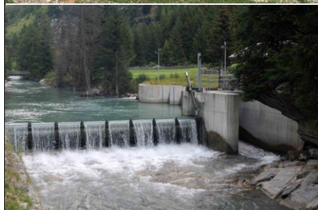
Temporary diversion structure made with loose bed sediments
