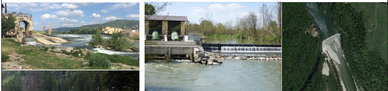
Top line: (left) abstraction weir with an abandoned mill; (centre) abstraction weir associated with an Archimedean screw hydropower plant; (right) Abstraction weir with movable gates.
