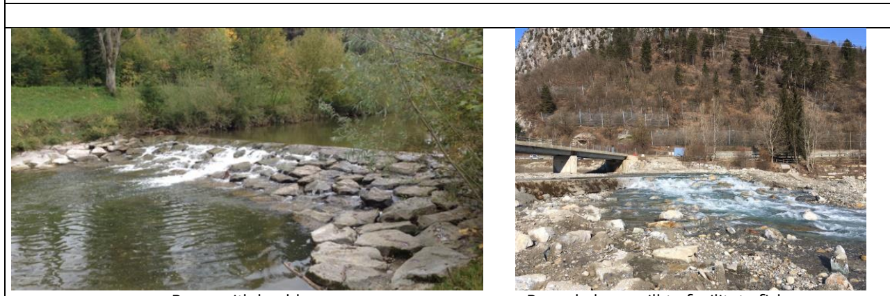
Ramp with boulders
