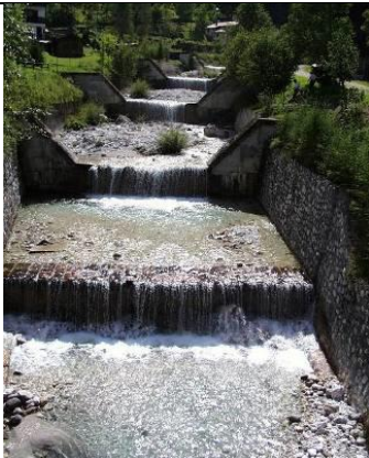
Series of consolidation weirs
