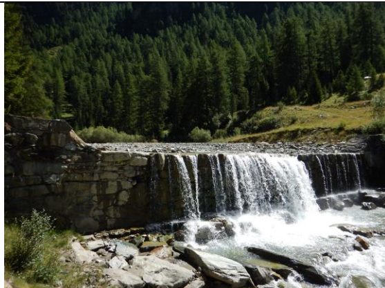
Consolidation weirs that are totally filled with sediments on the upstream side
