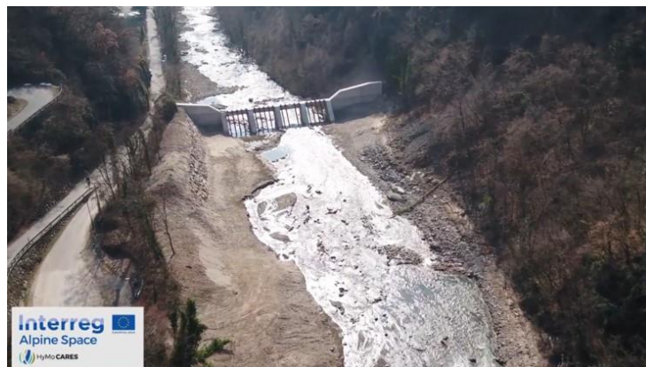
Selective retention weir with negligible impact on longitudinal connectivity for fish
