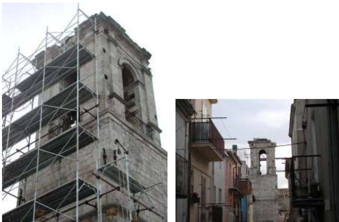
Figure 4.4. Partial collapse of the bell tower of the San Giacomo church in Santa Croce di Magliano
