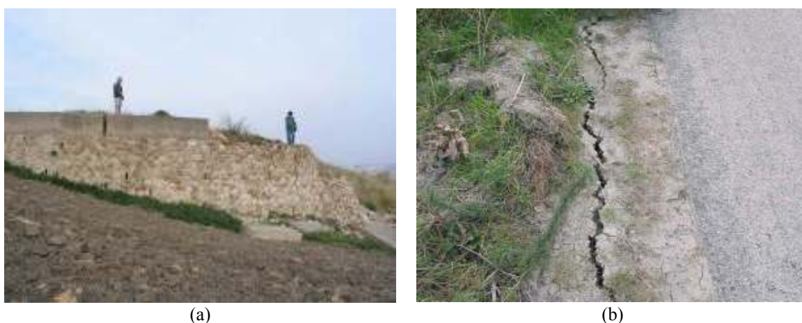
Figure 5.3. Roadside landslide (a) and roadside longitudinal crack (b) in the Vallepare area [INGV, 2002]
