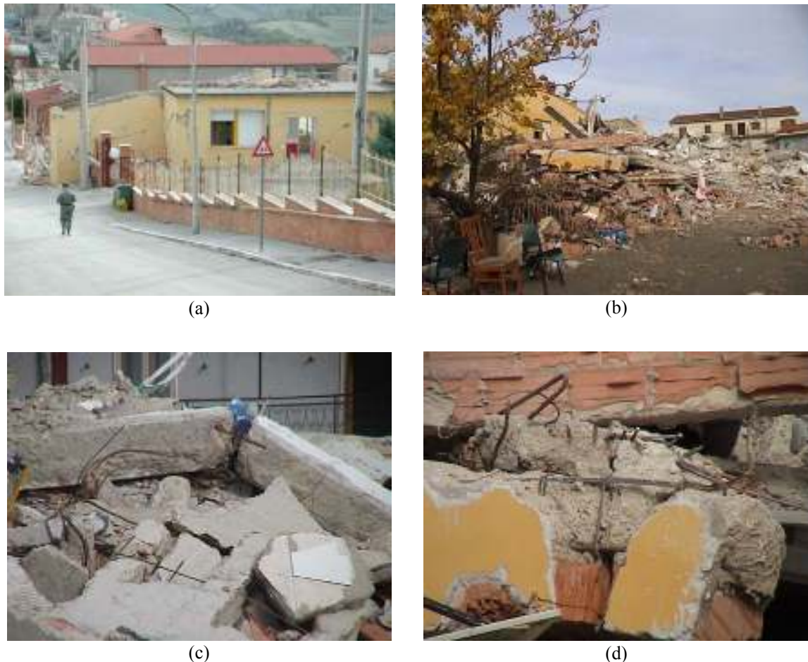
Figure 4.14. The collapsed school – ‘Scuola Francesco Jovine’ of San Giuliano Puglia: a) North view (a), South-west view (b), and details of collapsed RC members (c, d)
