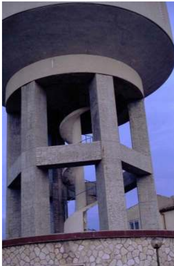
Figure 3.13. Reinforced concrete water tank in Morrone del Sannio
