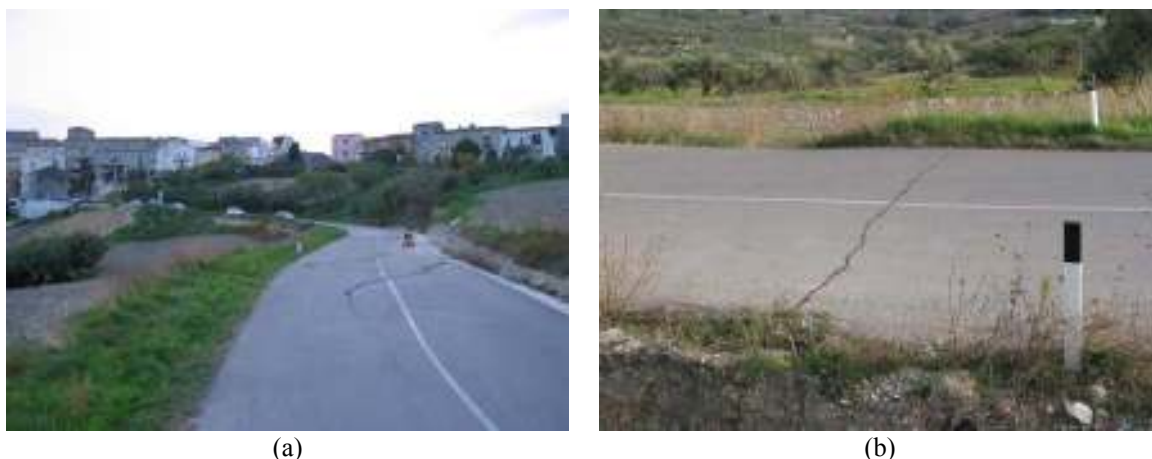
Figure 5.2. San Giuliano di Puglia: longitudinal (a) and transverse (b) cracks in the road [INGV, 2002]
