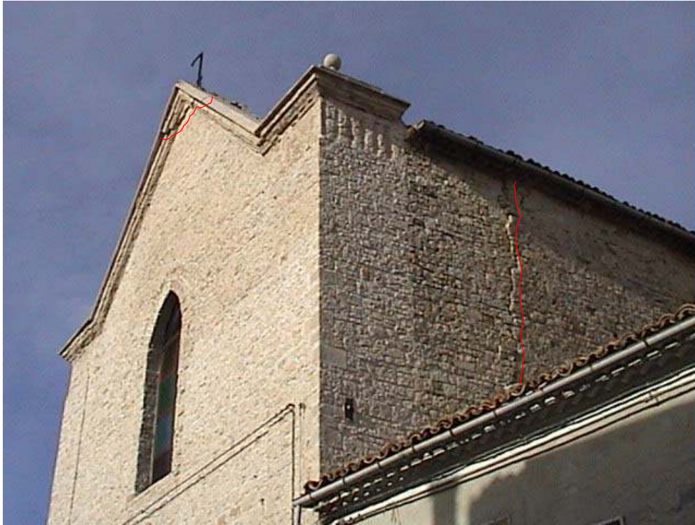
Figure 4.6. Old church in Ripabottoni, separation of the façade and overturning of spire
