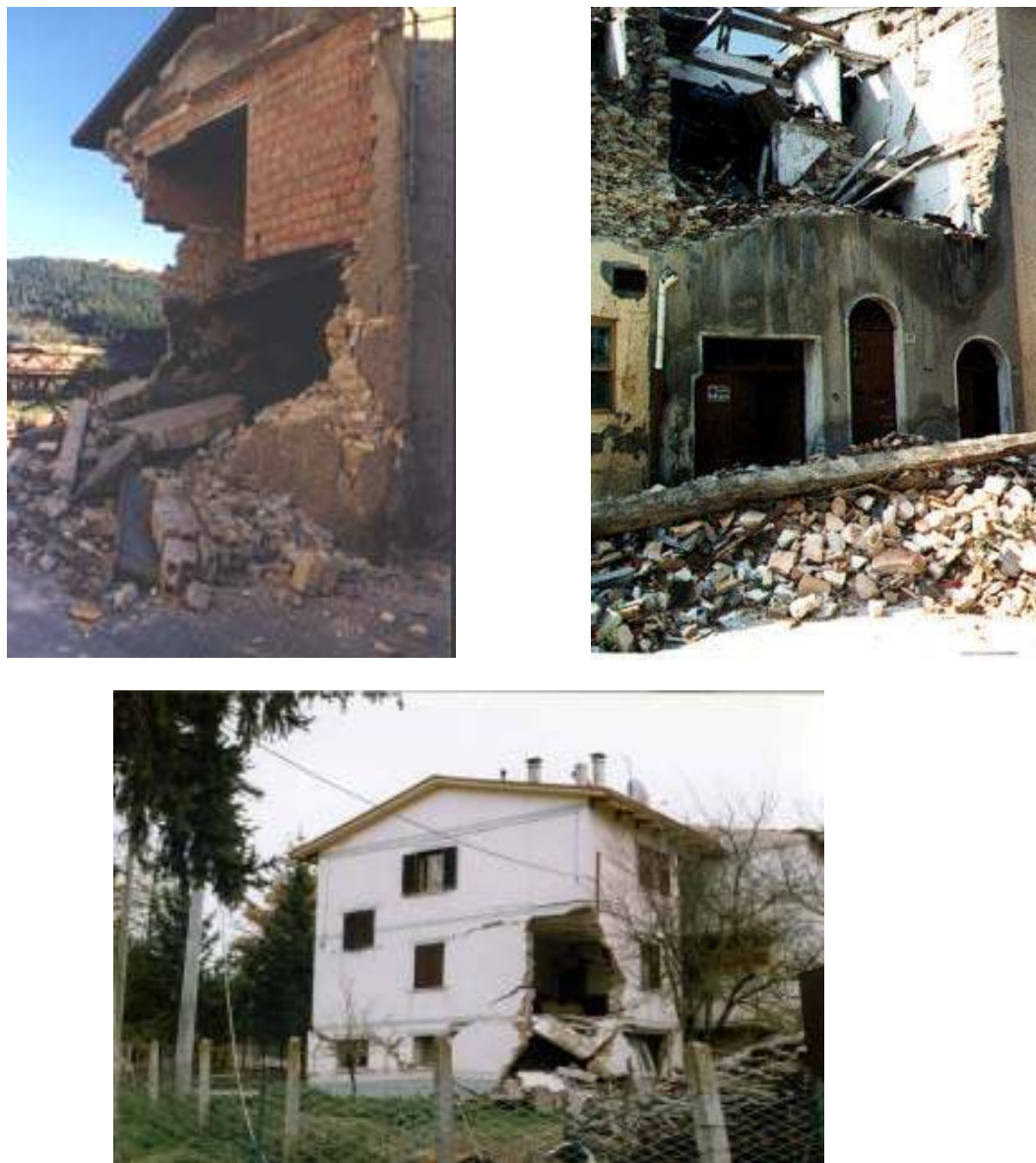
Figure 3.19. Damage of new and old masonry buildings in the Umbria-Marche earthquake [Primitally, 2002]
