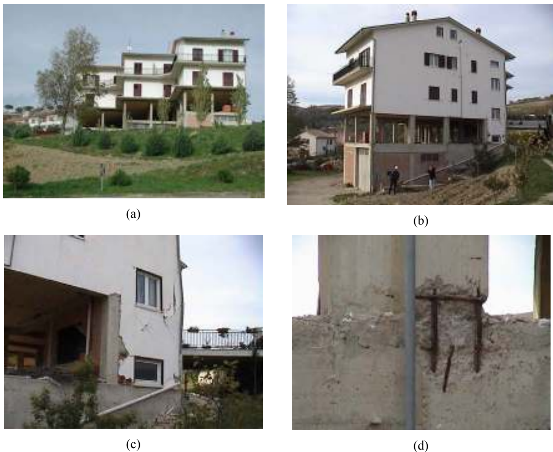
Figure 4.13. Reinforced concrete building in San Giuliano di Puglia, South view (a), East view (b), damage of infills (c) and damage at the base of a column (d)
