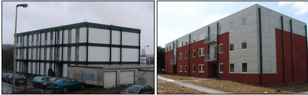
Figure 1: view of the apartment buildings before (left) and after (right) renovation
