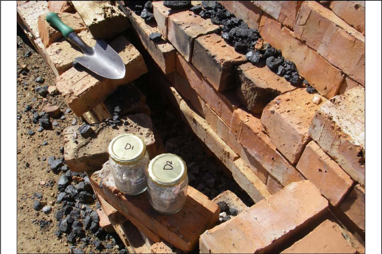
Figure 45: Detail SABK2, brick ingredient "fluff" (waste paper pulp)
