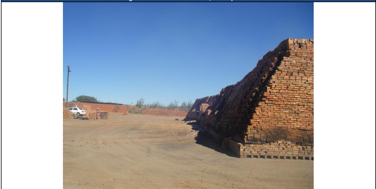
Figure 36: Detail SABK1 , clamp kilns
