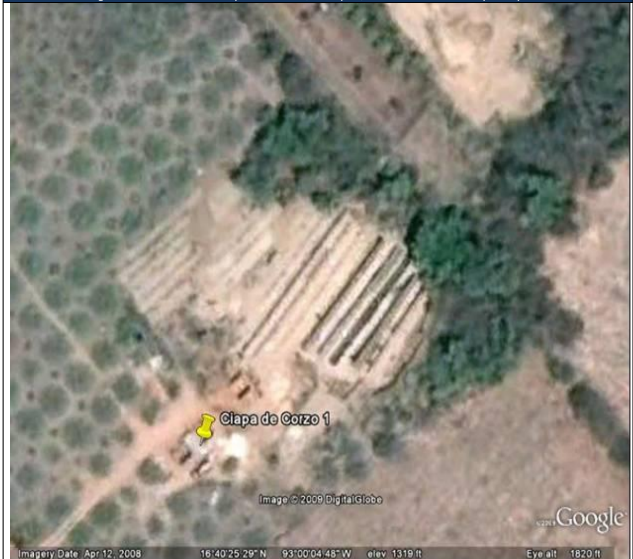
Figure 31: Location Chiapa de Corzo, Chiapas, waste oil fired temporary kiln
