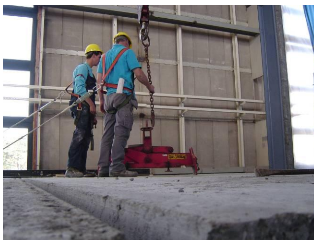
Example of working on height at JRC-IE for which a work permit is required.
