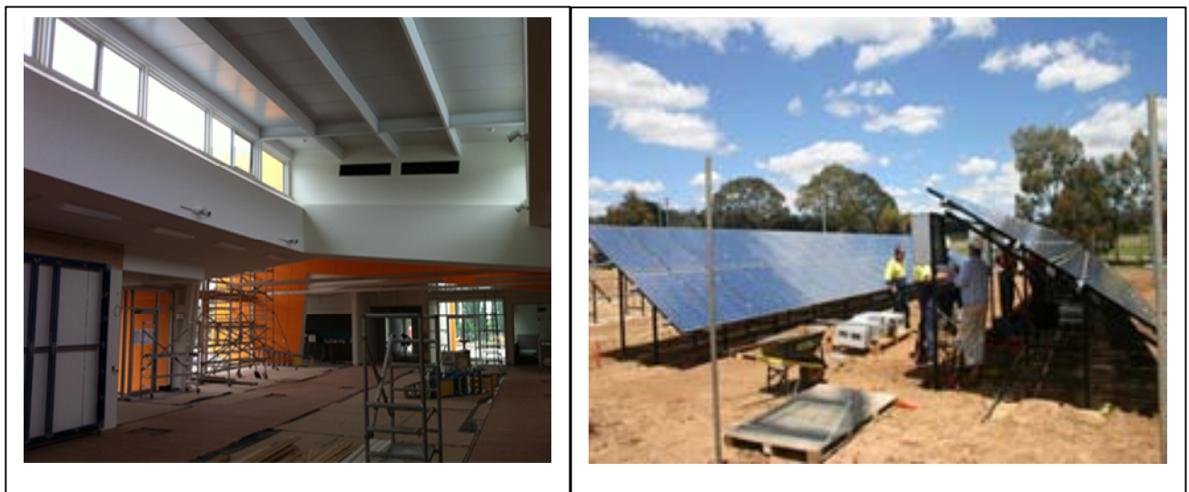
Figure 8: Flannery Centre – Gallery and Hub with timber floor plenum [L] and PV array [R]
