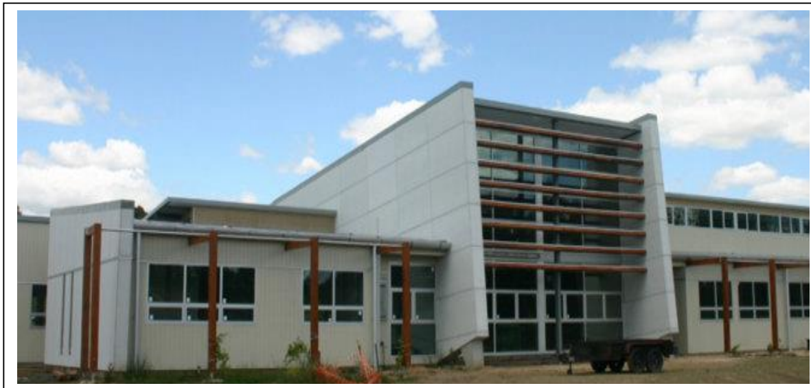
Figure 3: Flannery Centre – nearing completion December 2011
