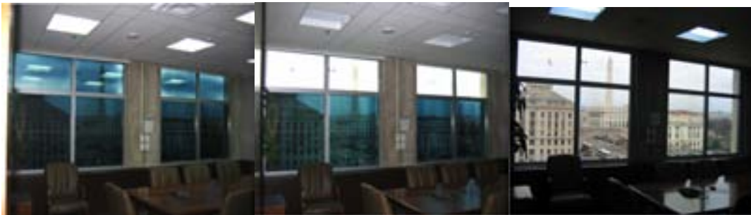
Figure 4. Photo sequence of conference room with electrochromic glass; with independently controlled lower view windows and upper daylight windows.
