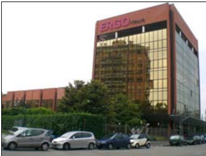
Figure 1 Case study building before energy retrofit
