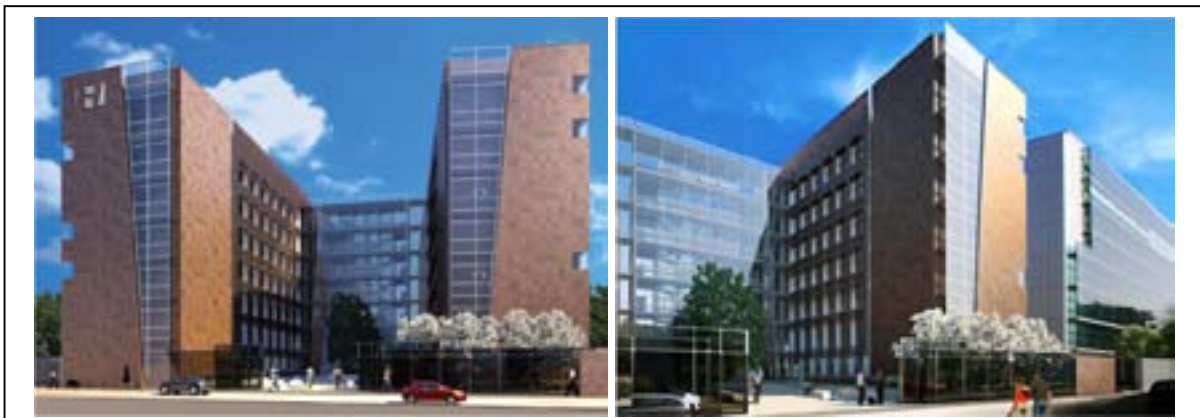
Figure 1 Views of the building.
