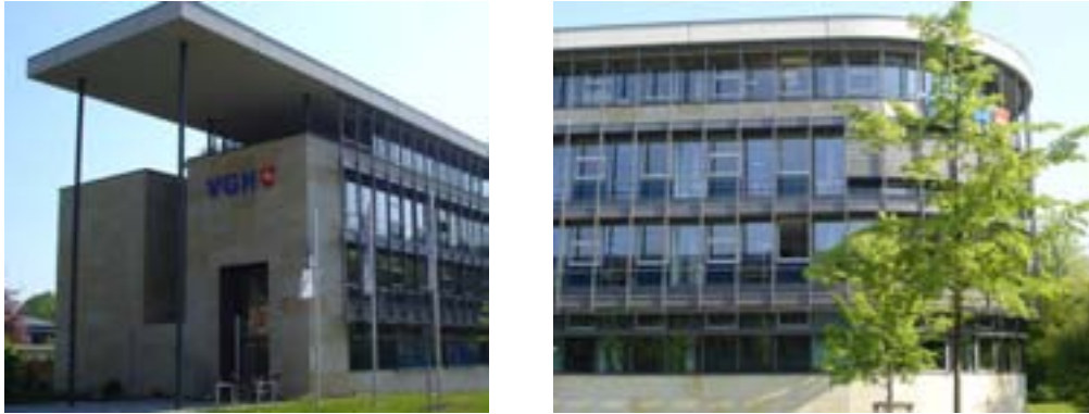
Figure 3 VGH-Lüneburg – view from west- (left) and from south side (right) [source: IGS]
