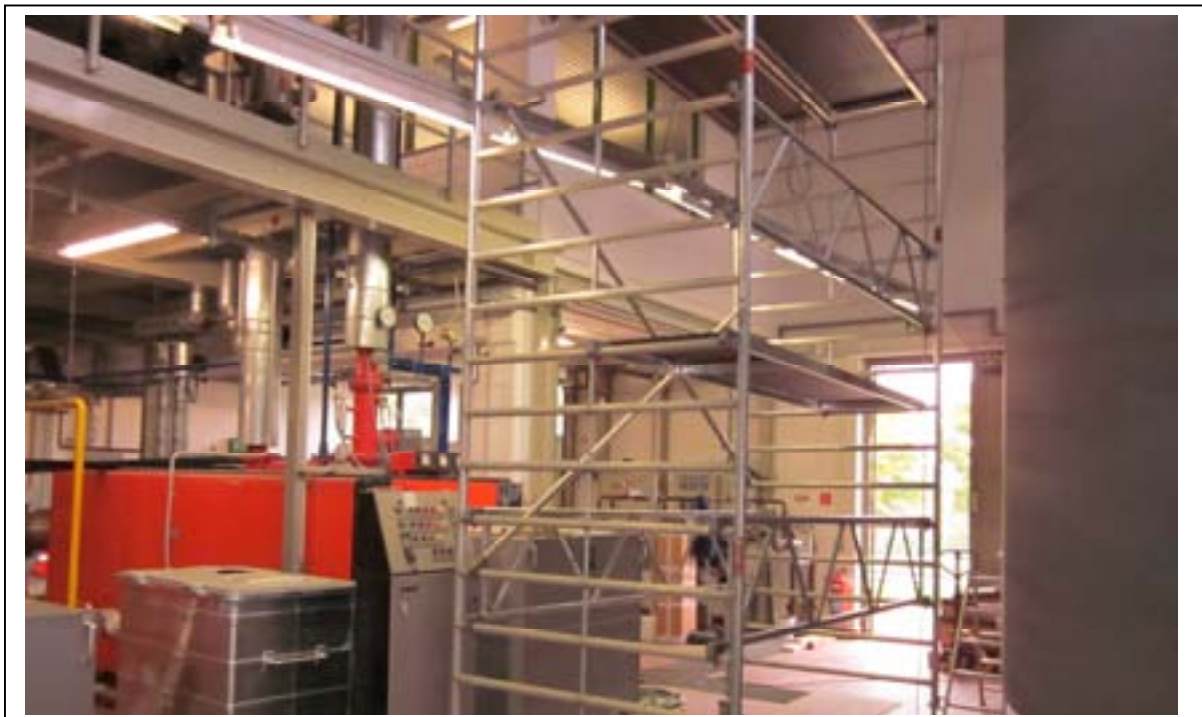
Final installation of a gas-fired CHP-unit (source: JCI)
