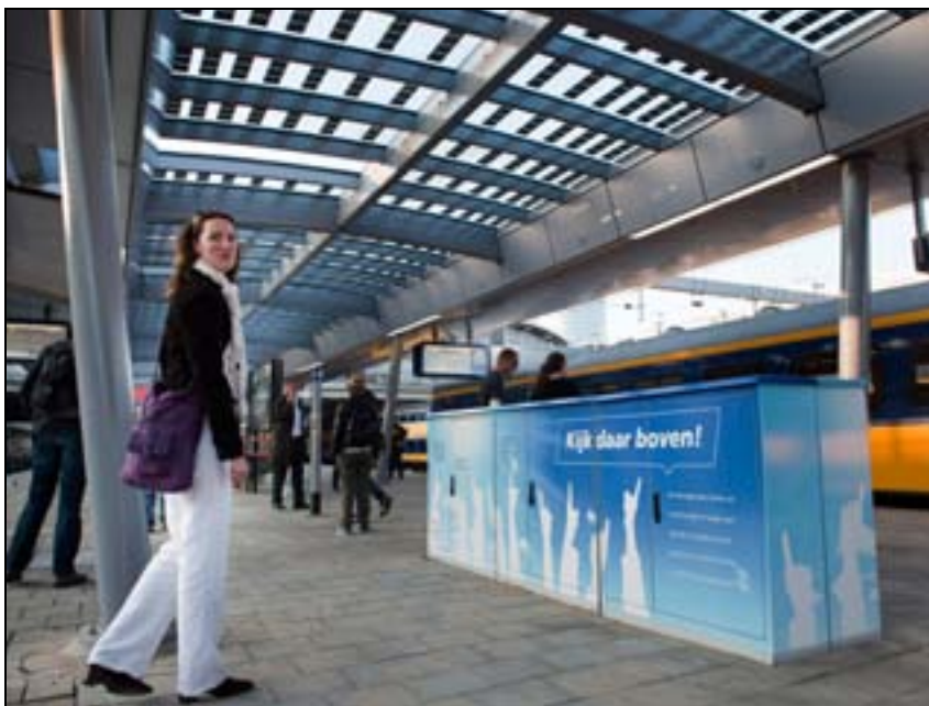
Figure 3 Utrecht Centraal Photo Voltaic panels within platform canopies
