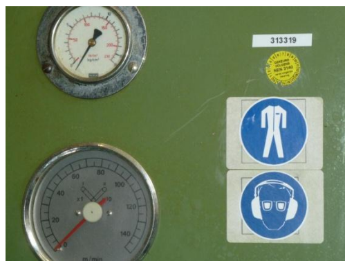
Inspection of electrical equipment
