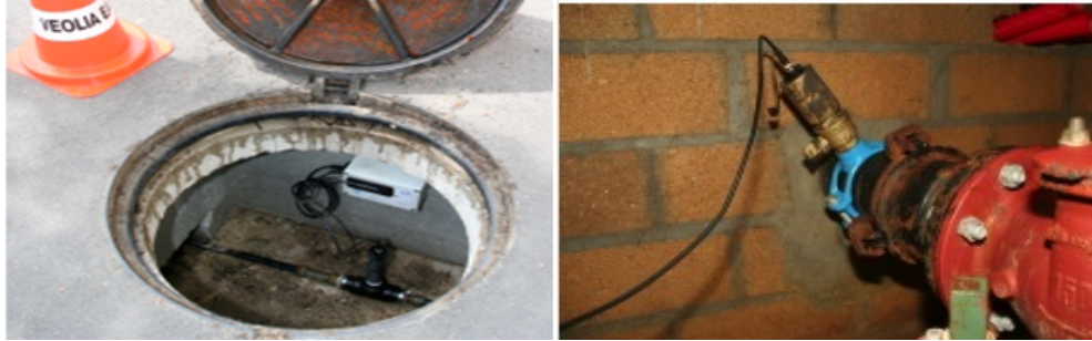
Figure 2. Kapta™ 3000 AC4 sensor installed in a distribution network [11]
