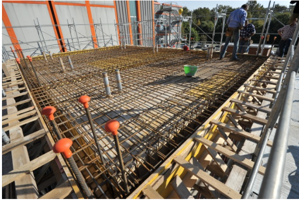
Figure 4.7 Slab reinforcement
