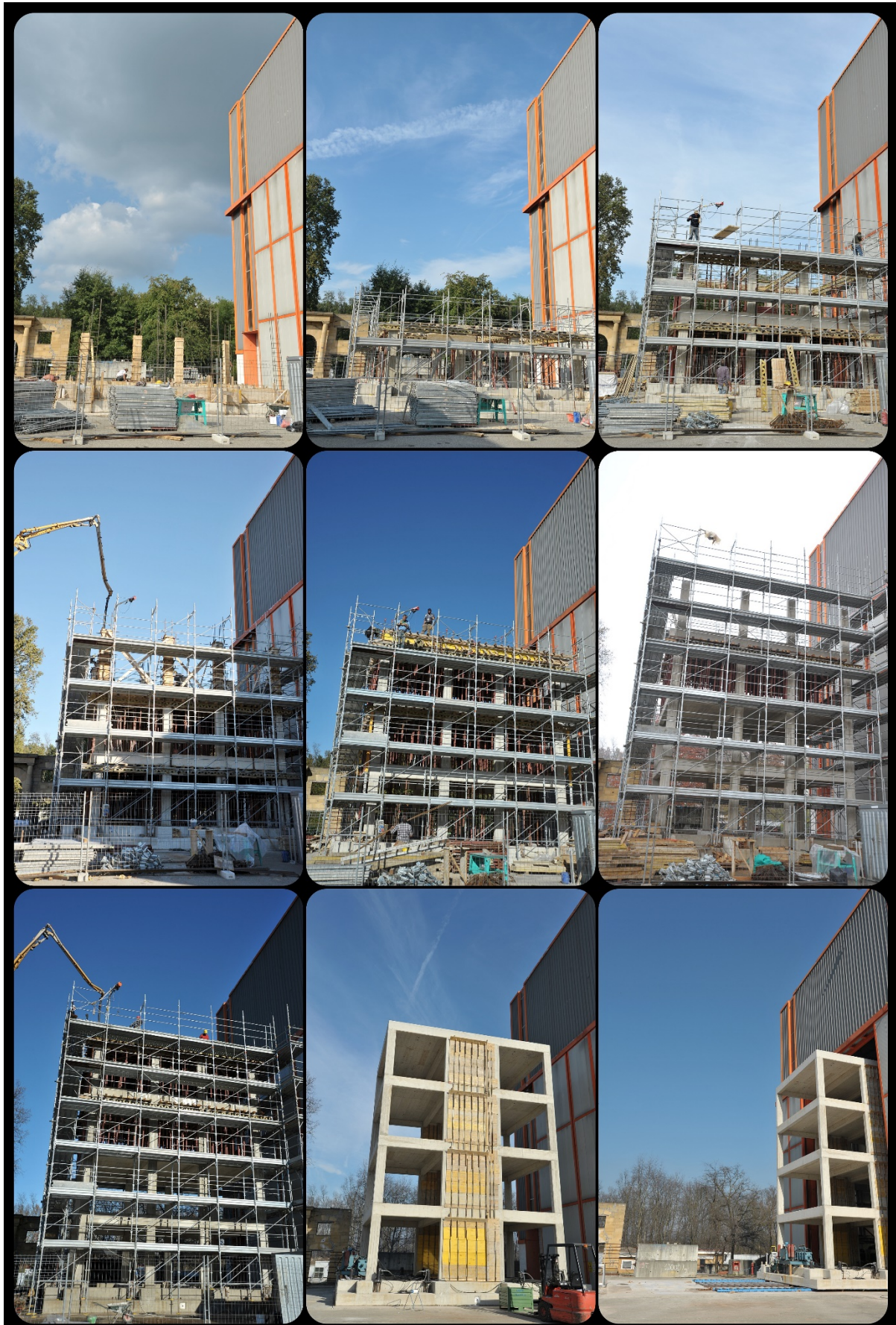
Figure 17 Construction phases of the SERFIN structure
