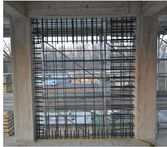
Figure 4.14 Dowels, starter bars and web reinf.
