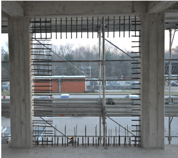
Figure 4.13 Dowels and starter bars
