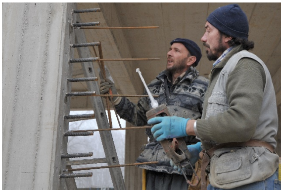
Figure 4.15 Installation of dowels and starter bars
