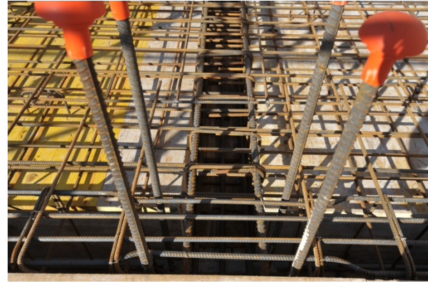
Figure 4.8 Reinforcement at a central beam
