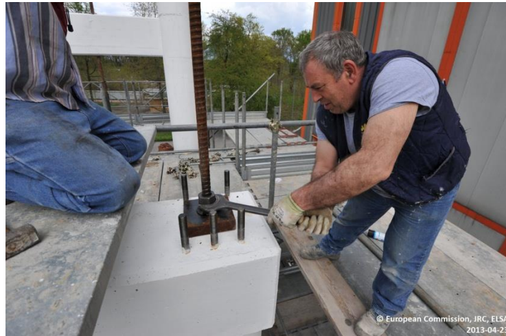
Figure A.5 Prestressing bars at top of the piers
