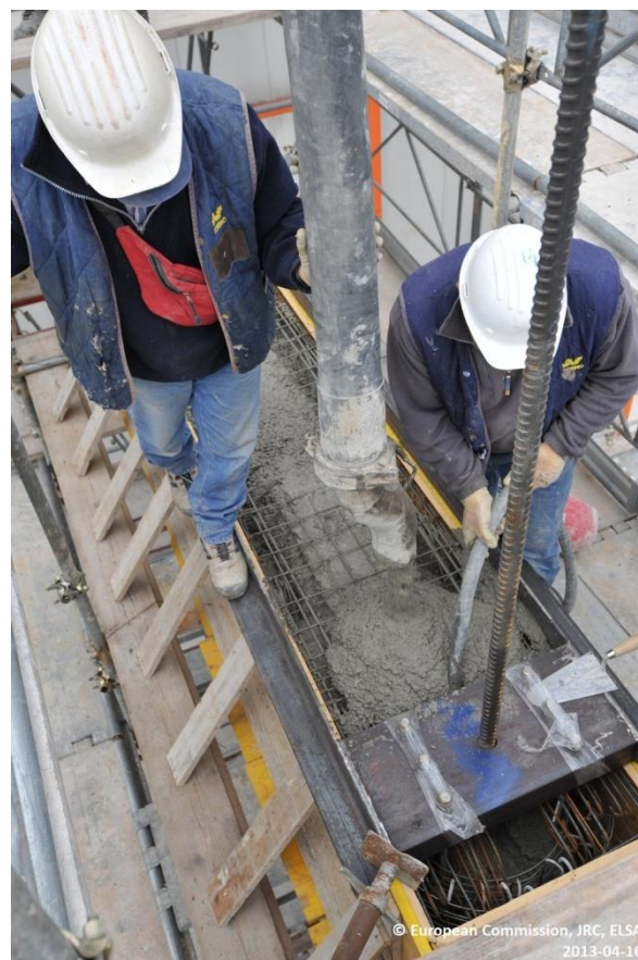
Figure A.4 Concrete pouring on beams
