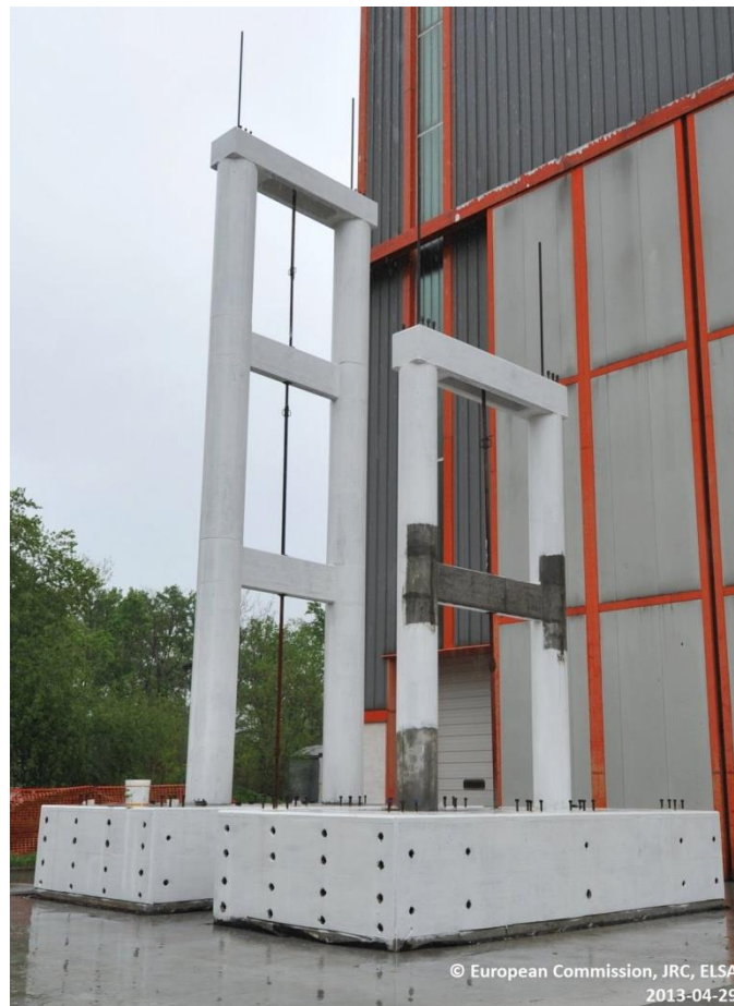
Figure A.6 Completed Construction piers
