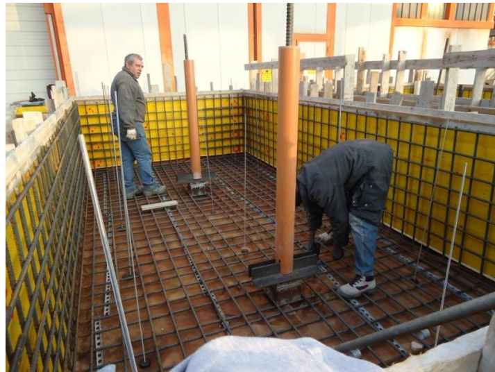
Figure A.1 Foundation Steel work
