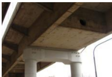
Figure 6.9 Rigid beams connecting the deck to the piers
