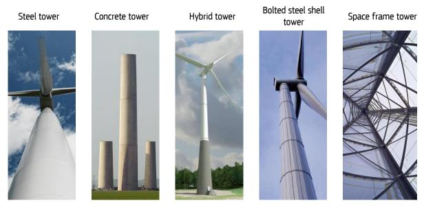
Figure 5: Different kinds of towers. Courtesy: Siemens, Acciona, GRI Renewable Industries and General Electric.
